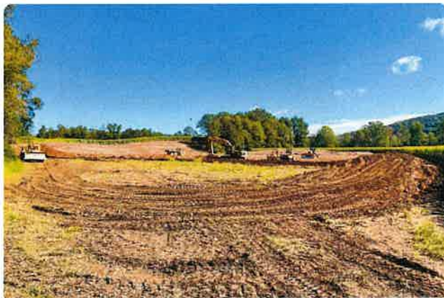
Hanehan Family Dairy, LLC Waste Storage project. Site work
