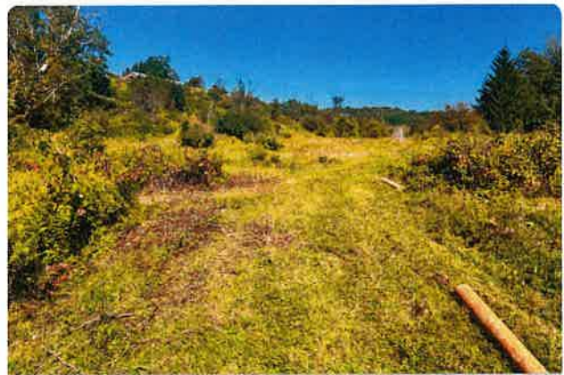
Hidden Falls Lands and Forestry- The contractor was busy yesterday laying out fence posts to begin pounding.
