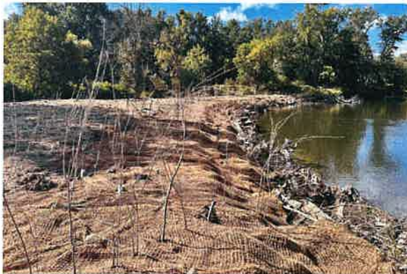
Nearly 2400 willow stakes and about 60 full length trees with root wads attached were used for the project.
