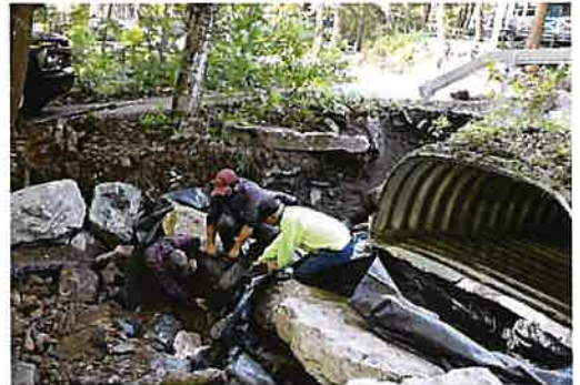
Installing filter fabric at Warner Brook.
