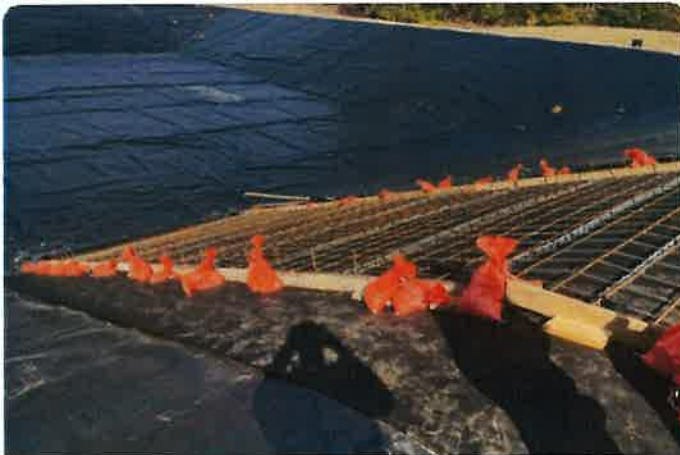
Hanehan Family Dairy, LLC Waste Storage project. Pictured above is tied rebar and forms for the concrete ramp installation.
