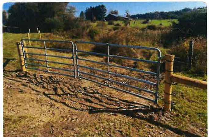
During the week of September 29th, the contractor completed the fencing project for Hidden Falls Lands and Forestry, above is double 8-foot gate opening for a livestock crossing.
