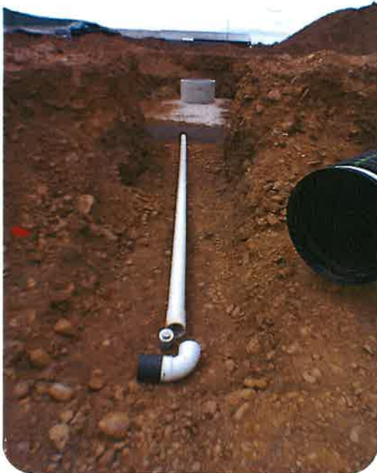
Photo left: Bunk Silo Project – Mount Upton – This is a 3,000-gallon precast pump tank for the low flow leachate. The low flow leachate will be pumped to the concrete manure storage across the road.
