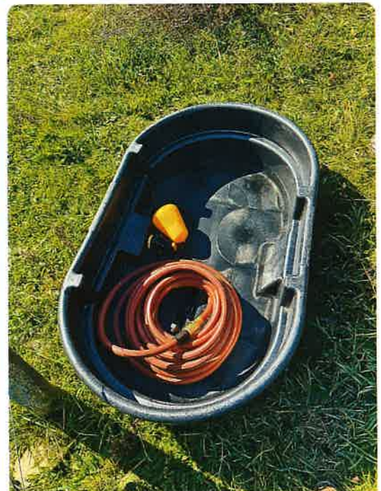
The farm installed eight watering troughs, each equipped with 50 feet of heavy-duty garden hose, and a Jobe Float valve.
