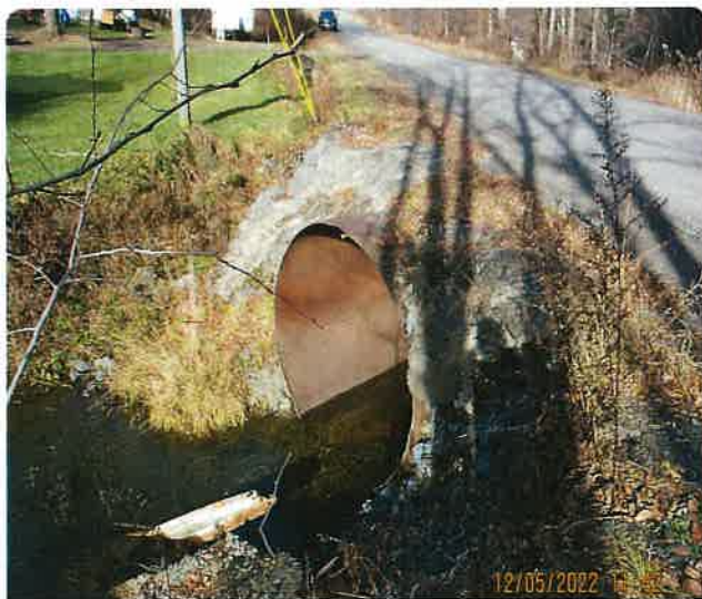
Original steel culvert outlet
