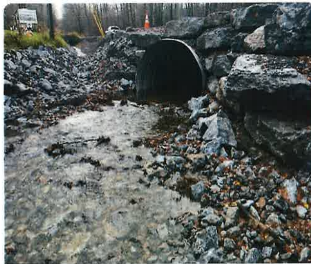
You can see the fully finished outlet of the pipe arch, headwall, and additional stabilization measures to handle high storm velocities.
